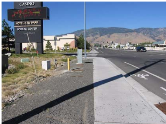
Existing sidewalk on Hwy 50 looking west
