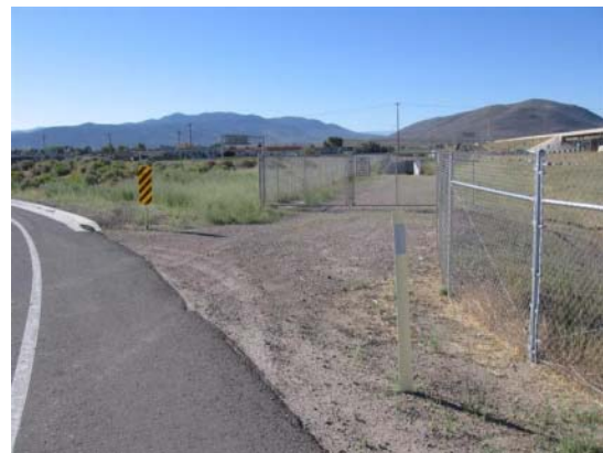
NDOT maintenance access
