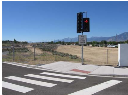
Looking south from existing signal at Fairview Drive
